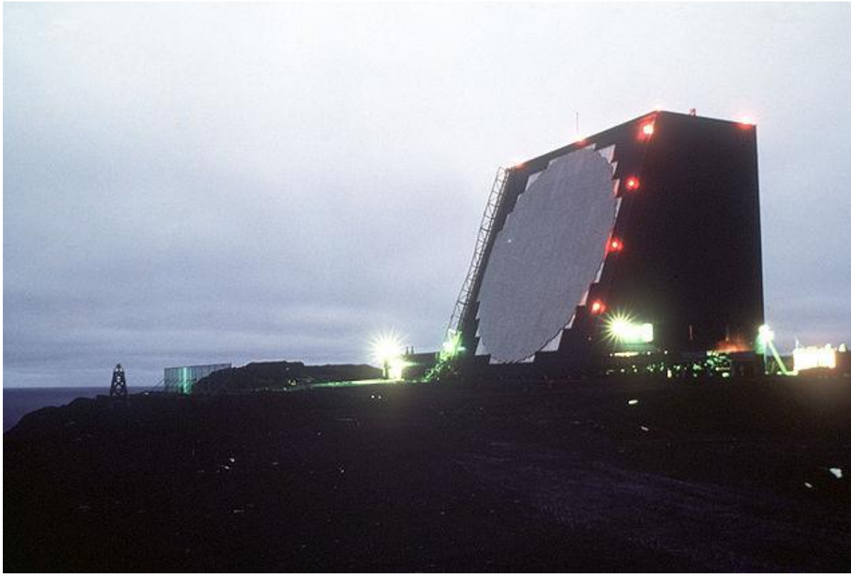
COBRA DANE, an intelligence-gathering phased array radar, Shemya Air Force Base, Alaska, adopted from Wikipedia
